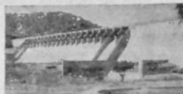
Building of irrigation and multipurpose dam
