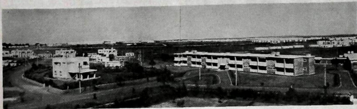
Bhopal Heavy Electricals, for which Associated Electrical Industries is to be expanded in two phases, with British aid as indicated by Lord Chandos during his visit last year.
